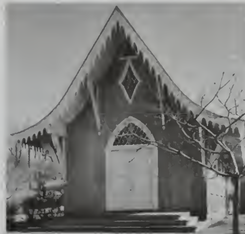
Gothic Revival style bargeboard on the New York Yacht Club House (currently in Mystic, Conn., U.S.), by Alexander Jackson Davis, 1846
